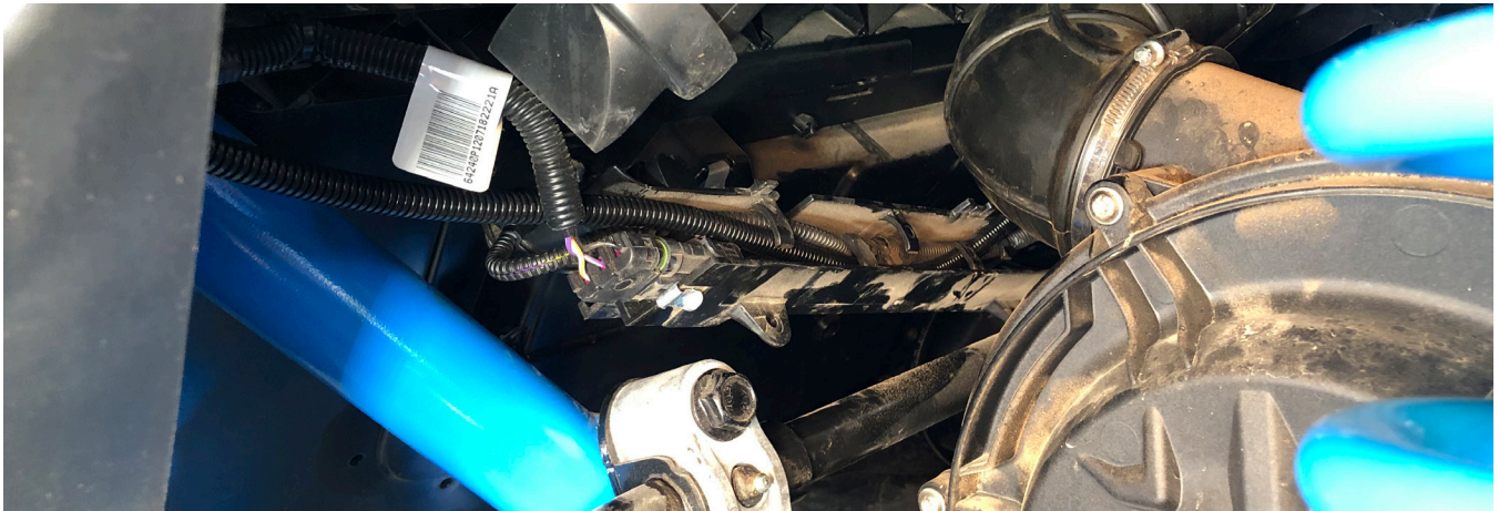
Figure 9b: Shows harness being routed along the left-side cable channel located between the cab and the motor.
